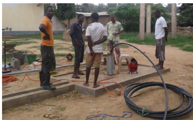
Figure 27: Carrying out pumping test on a selected borehole
