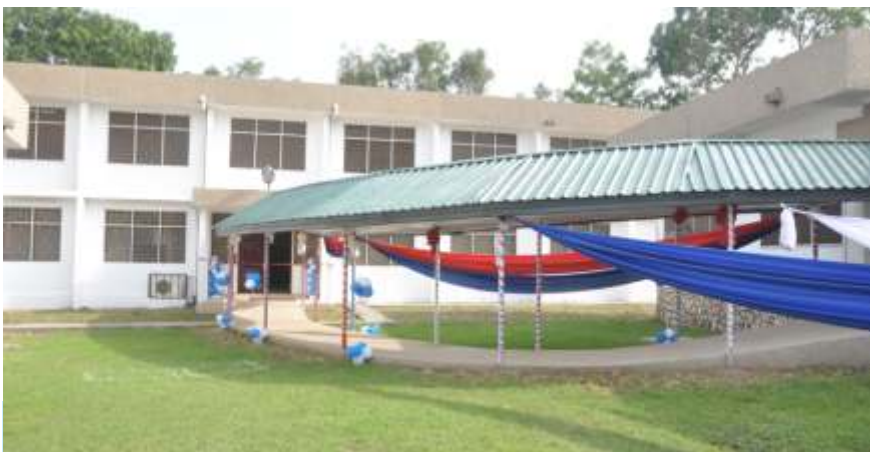
Walkway to the New Office Block
