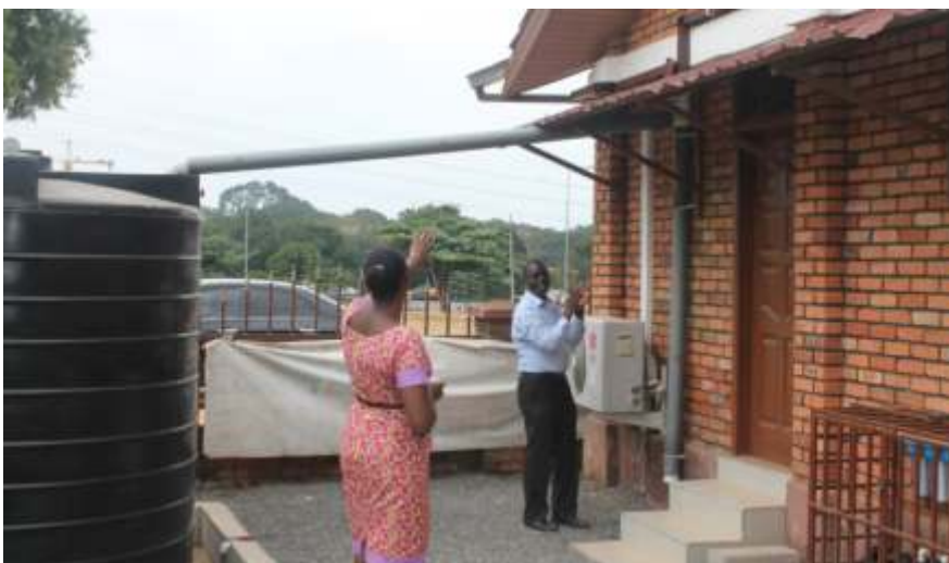
A member of the research team explaining the operation of the RWH system to a beneficiary of the project
